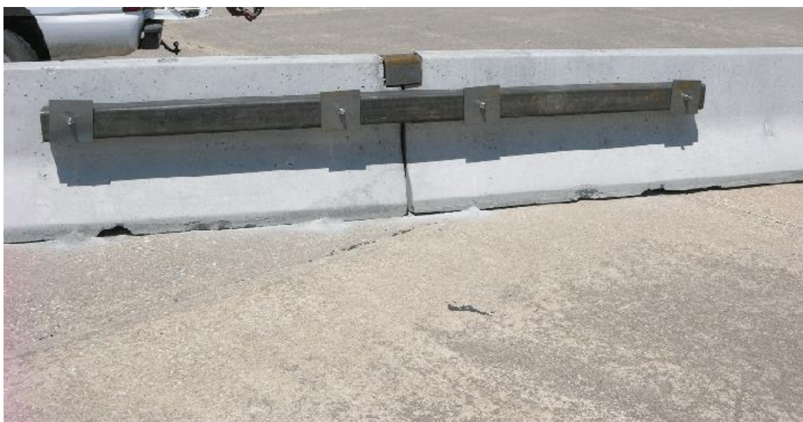
Figure 25. NYSDOT Box-Beam Stiffener System [29]
