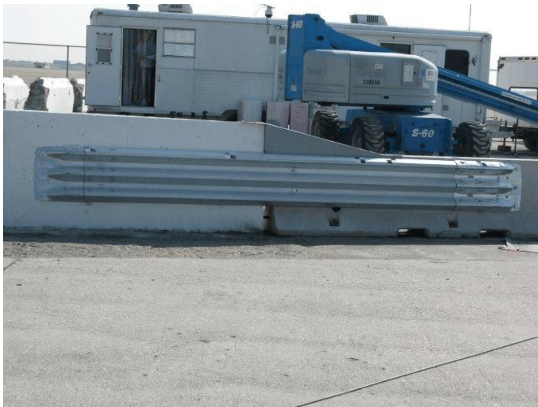
Figure 11. Transition from PCB to Permanent Concrete Barrier [2]
