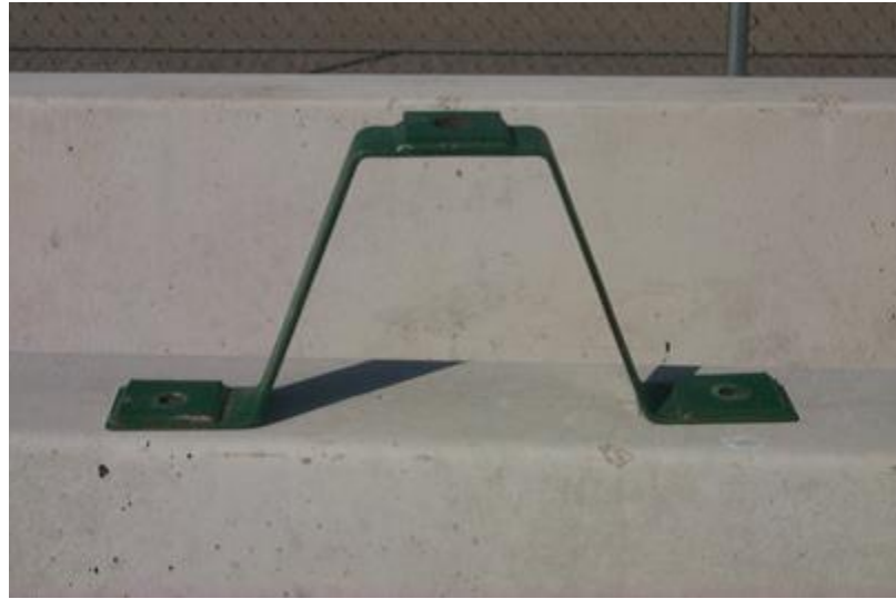
Figure 7. Steel Tie-Down Strap [12]
