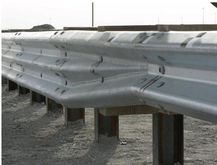
Figure 19. MGS Stiffness Transition with Asymmetrical Element [21]
