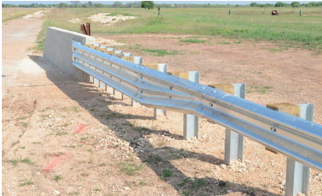
Figure 20. Thrie Beam Transition without Curb [23]
