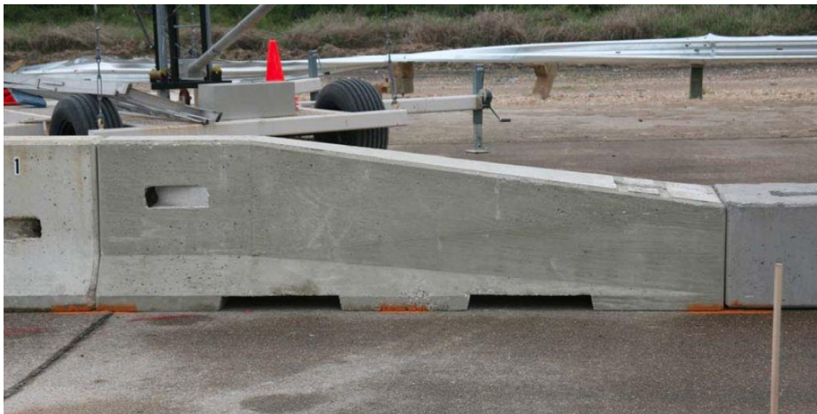
Figure 22. Low-Profile to F-Shape Transition Barrier Segment [25]
